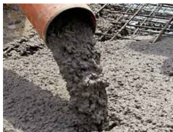
FIGURE 1.4 – Fabrication de béton
